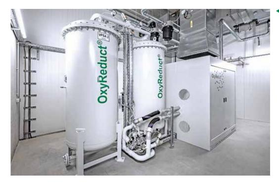
OxyReduct-V-Line® systems generate the nitrogen required for oxygen reduction from the ambient air and introduce it into the protected area.
