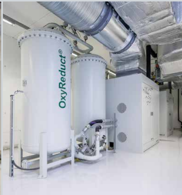
The two OxyReduct® systems get their nitrogen from the ambient air. This nitrogen is then fed into the protected area through a distributor pipe network.
