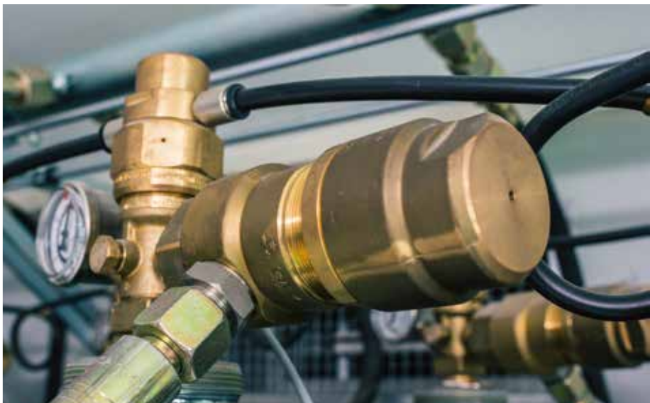
Flow regulator for soft flooding
