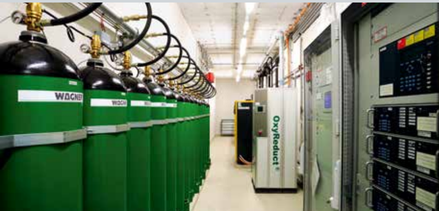
The OxyReduct® fire prevention system with fast reduction.
