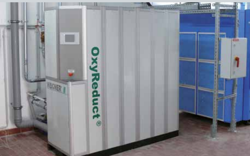
Nitrogen generator (left) for the generation of nitrogen, one of the core components of an OxyReduct® fire prevention system.
