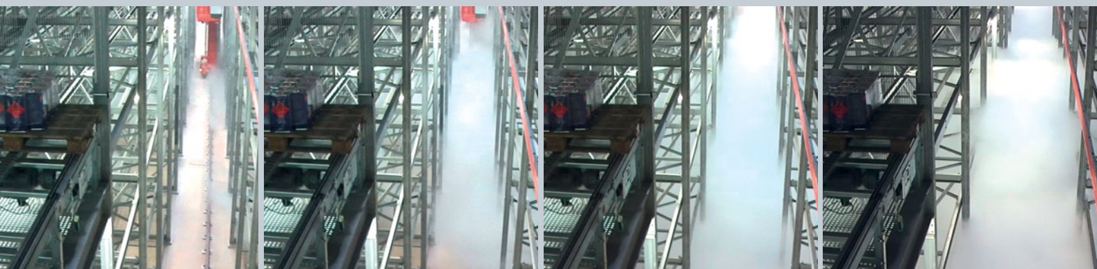
▲ The FirExting® inert gas extinguishing system is controlled by a flame detector and responds to alarms by creating a CO 2 extinguishing fog of up to five metres in height.
