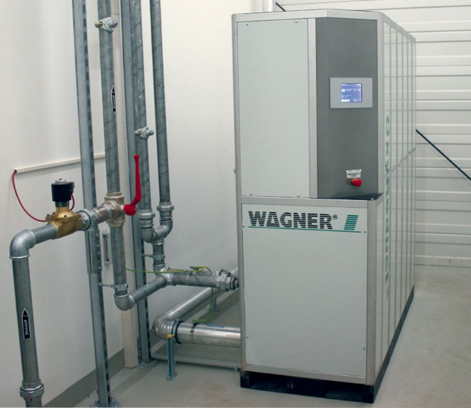
▲ An OxyReduct® system provides fire prevention.
