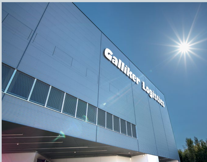
▼ Galliker stores food, non-food and pharmaceutical products in around 37,000 pallet spaces at its logistics centre.
