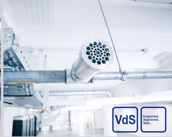
▲ Extinguishing nozzles with special sound absorbers.
