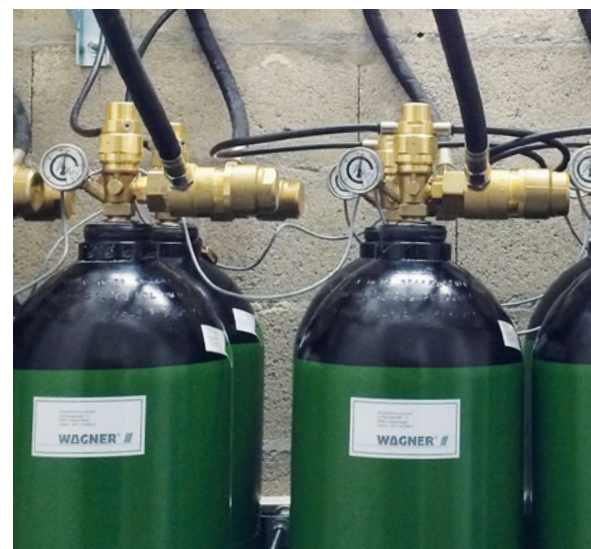
▼ Soft flooding: Extinguishing cylinders are equipped with flow regulators.
