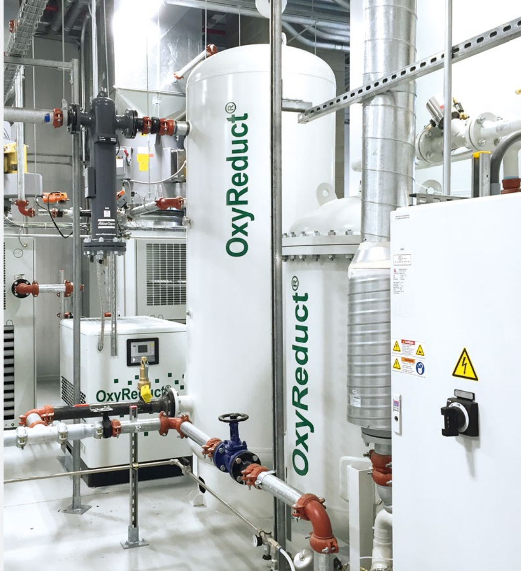
▲ The Preferred Freezer Services warehouse has become the first building in the USA to use WAGNER's OxyReduct® system for fire prevention.
