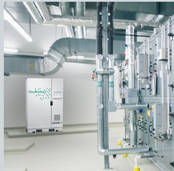
▲ The OxyReduce® fire prevention system lowers room atmospheric oxygen level from 20.9 to 15.9 vol.%.
