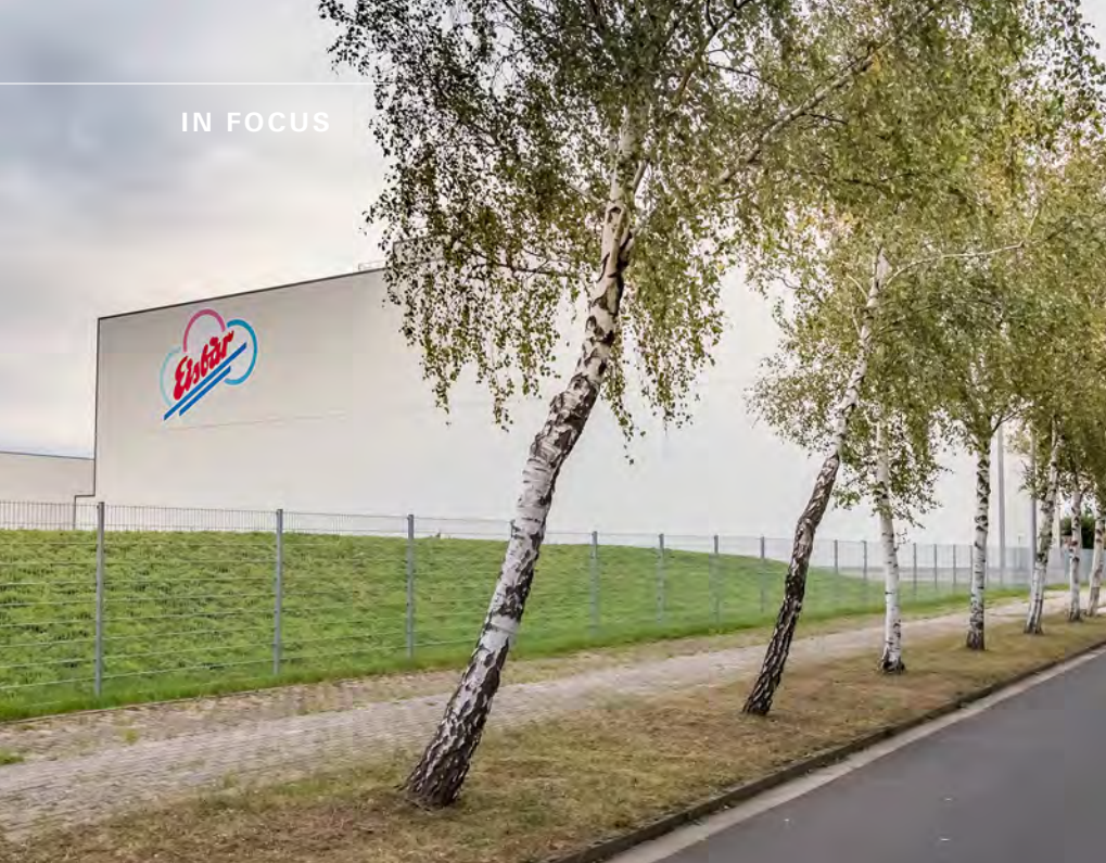
▲ Eisbär Eis: An OxyReduct® system with VPSA technology protects the deep freeze complex.
