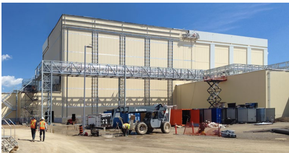
▲ The Dr. Oetker deep-freeze high-bay warehouse during construction phase
