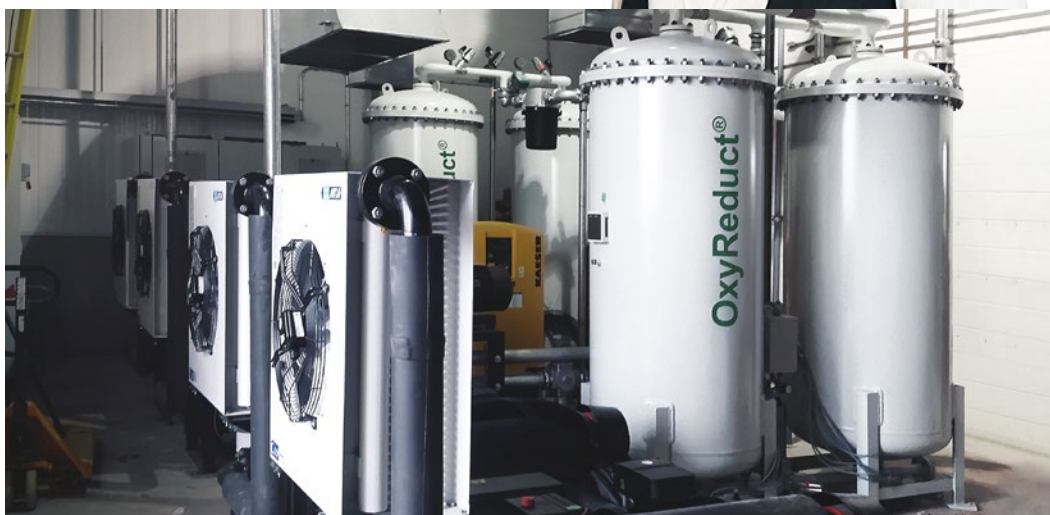
▲ The WAGNER system constructors had around six months to design and set up the VPSA system specifically for the Canadian market
