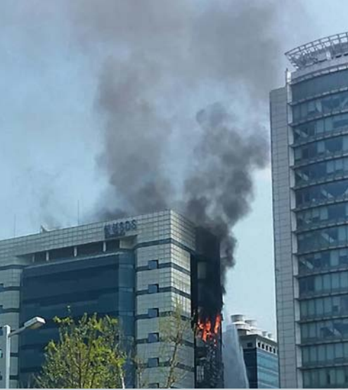
▲ On 20/04/2014 a fire broke out on the fourth floor of the Samsung data centre in the South Korean city of Gwacheon. The incident resulted in a breakdown of Samsung services. Smart phones, tablets, smart TVs with smart hub, credit card services and other devices around the world could not be used for hours
