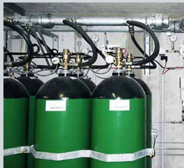
► A FirExting® gas extinguishing system from WAGNER protects the valuable exhibits in the wet collection
